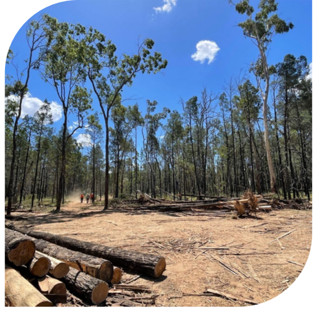
Example of already cleared landing
