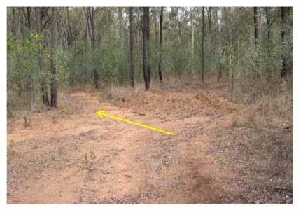
Figure 19: Water bar with side drain on a snig track
