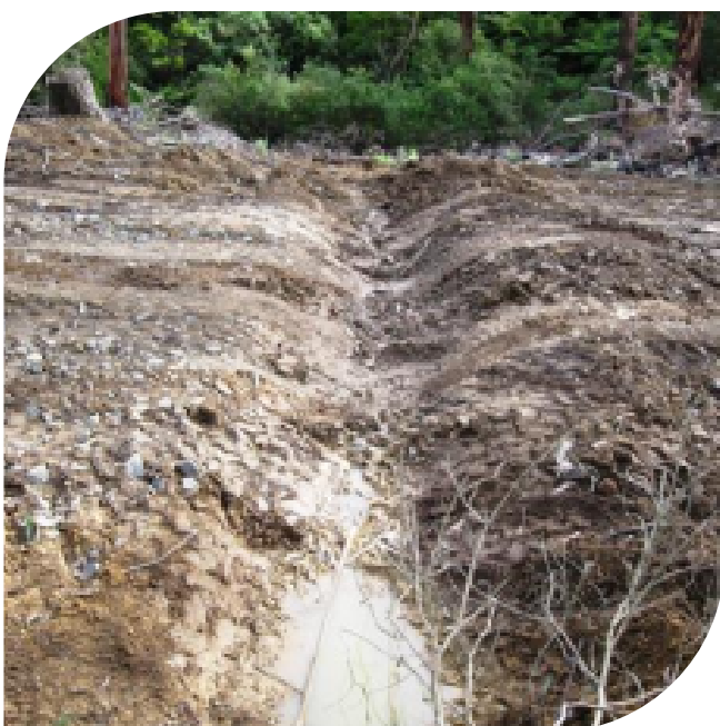
Cross Drain Source: HVP, 2022
