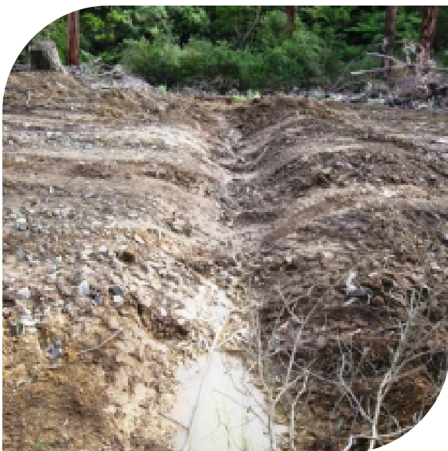
Cross Drain Source: HVP, 2022
